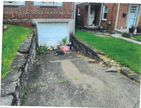
Solid waste in the driveway. 5/26/2022 AJL
