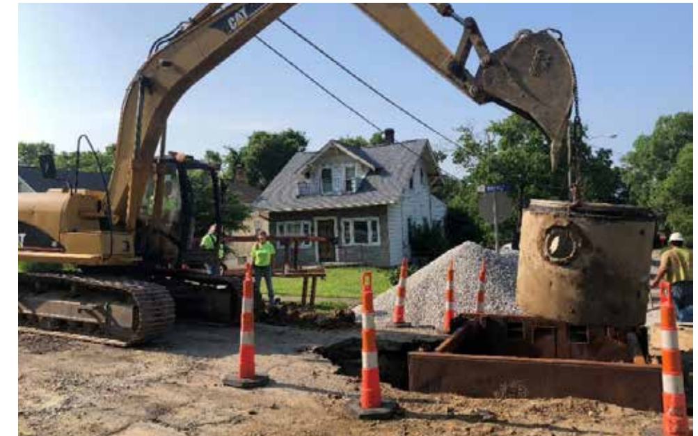
Construction on Maphet Lane
