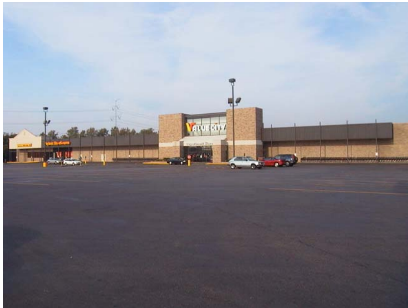
The Value City site is a highly visible, yet underutilized site and could support additional development.
