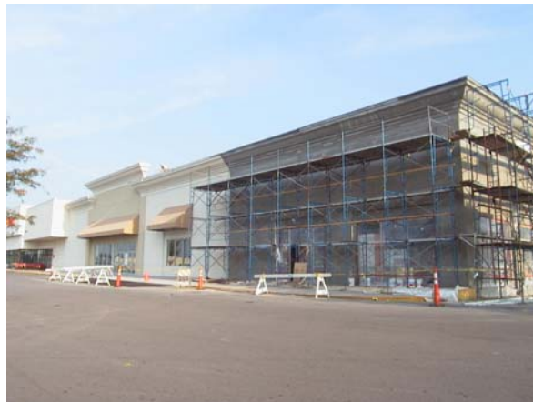
The new façade for AJ Wright, in Ridgewater Plaza, is under construction.
